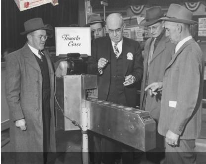
Model X (1940s). A total of 121 units were sold. Back then, canned tomatoes contained a hard, green core that required removal.
